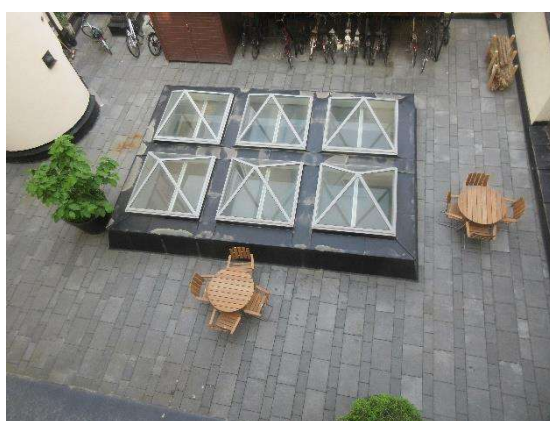
Stora innergårdens lanternin
